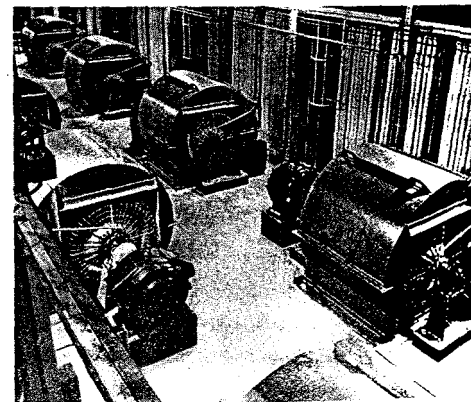
Fan room, with bag filters in background
